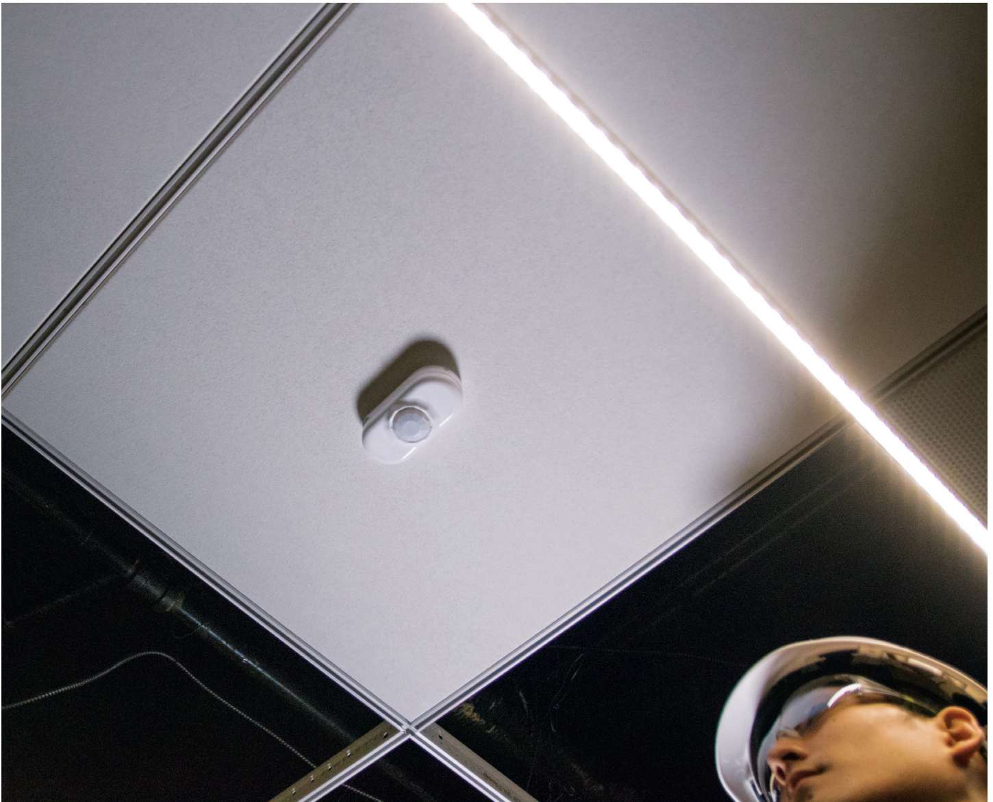
An Audacy Ceiling-Mount Motion Sensor controls the T-Bar LED™ by JLC-Tech light fixture in this installation.
